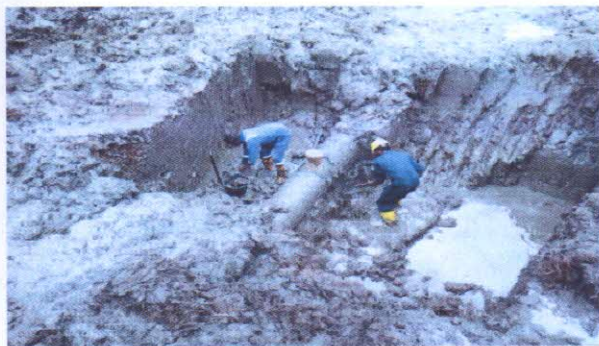
REPAIR WORK DONE BY NAOC REPAIR TEAM
