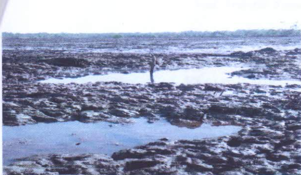
SPILL POINT BEFORE EXCAVATION
